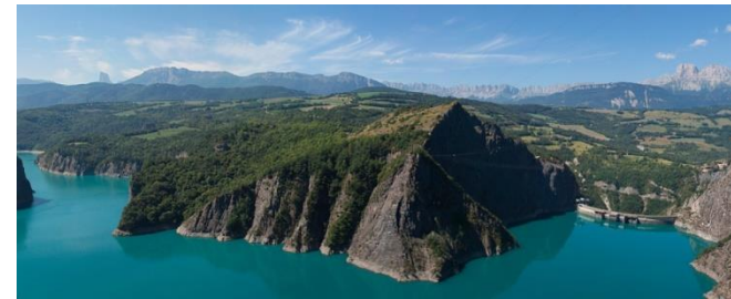
Dam in Monteynard (Drac)
