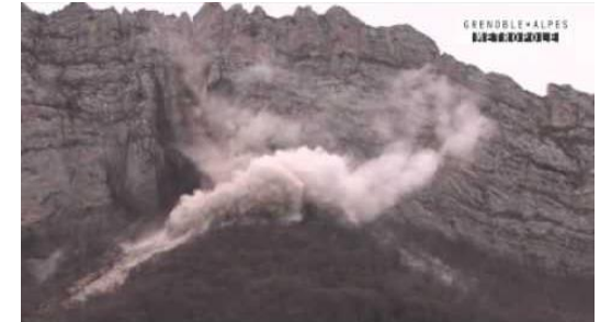
Crumbling of Ripaillère, 2011
